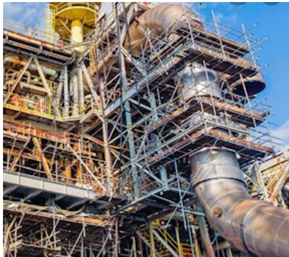
Figure 33 Tube and Coupler Scaffold
