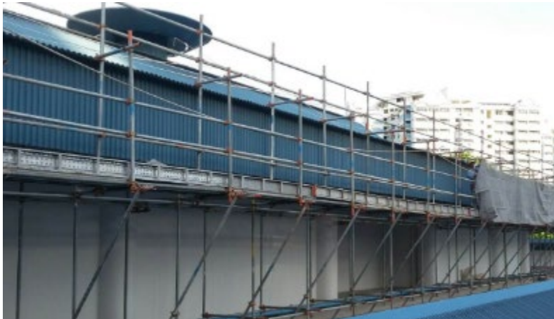
Figure 32 Cantilever Scaffold
